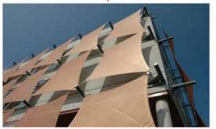
The use of tensile structure in windows minimizing the impact of the east sun during the day, it not only mitigates heat but also contributes to maintaining a comfortable temperature within the building. This innovative approach to window design reflects our commitment to energy efficiency and creating a more sustainable and comfortable learning environment for students.
