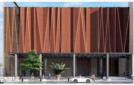
Aluminum perforated sheets have been installed on the frontage of the building. This designchoice not only adds an attractive and madern aesthetic to the building's exterior but also servespractical purposes such as shading and ventilation control while allowing for natural light to filter through.
